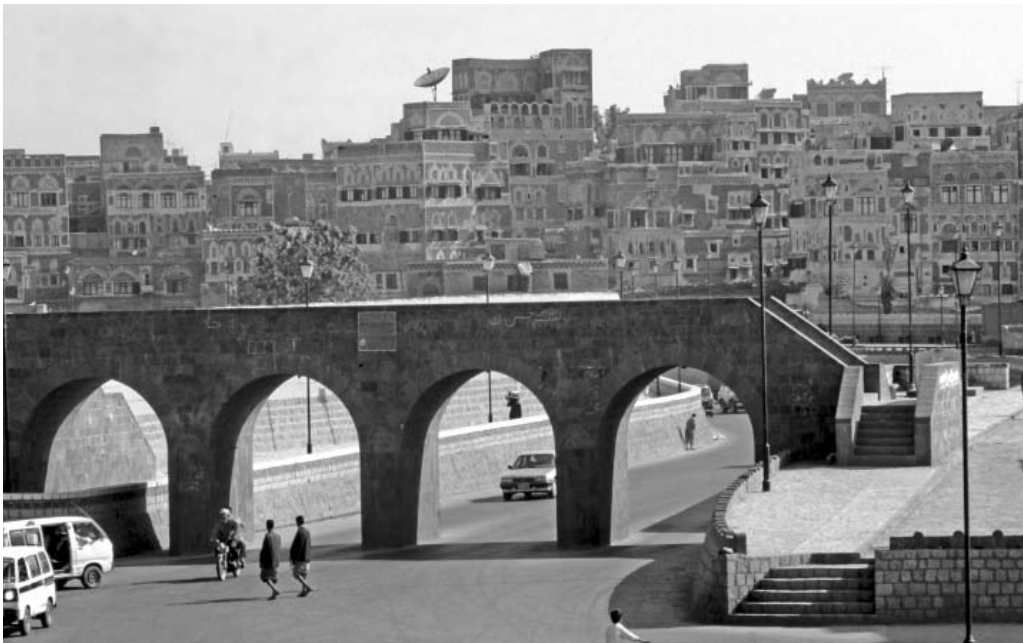
Photo 3.7: Roadway/flood channel Yemen. Source: Bill Lyons/World Bank
