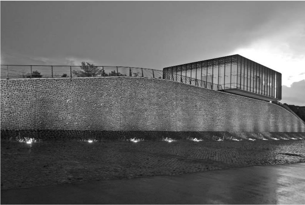
Photo 7.1: Pumping station in Cologne. Source: Peter Jost, pj-photography.de
