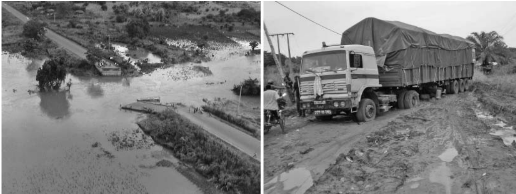
Photos 2.2 and 2.3: Roads destroyed in Togo, 2008. Source: Ayeva 2011
