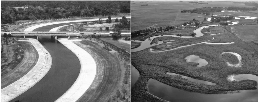
Photos 3.2: Highly channelized red Rouge River Dearbon for flood control purposes source USACE; Photo 3.3 Riverine Wetlands in Northwest Iowa, Source Lynn Betts.
