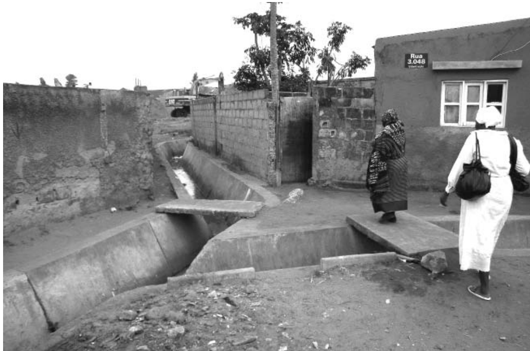
Photo 7.2: Drainage in Maputo Bairro Urbanização, Well-functioning drainage is very important for preventing that sanitary systems overflow during heavy rainfalls. Source Sustainable sanitation/Åse Johannessen
